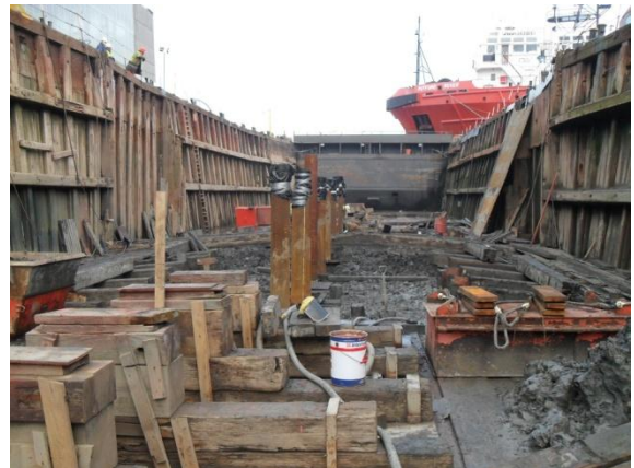
Installed bearing piles
