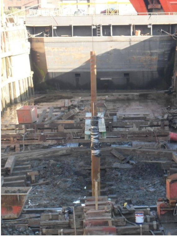
Installed bearing piles
