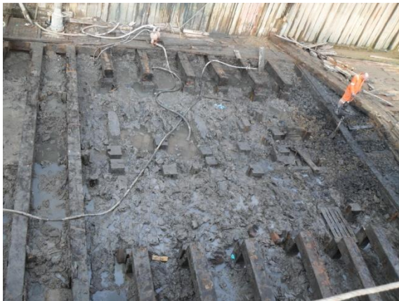
Area ready to install new bearing piles
