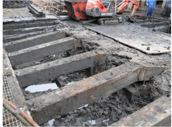
Snapped 12"x12" horizontal bearing beams
