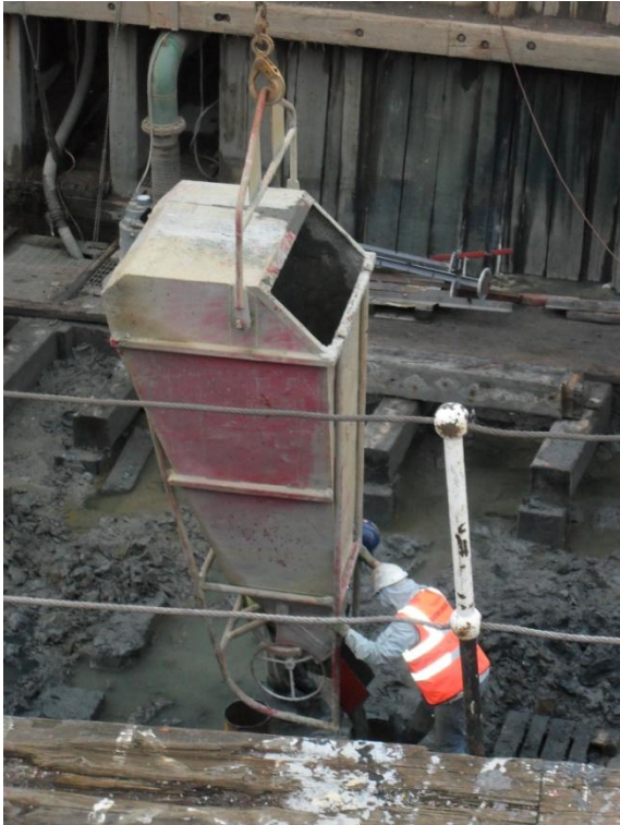
Treming concrete using our 2m 3 skip
