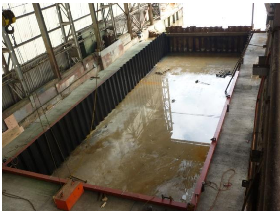
Completed concrete inside dock with cofferdam wall still in place
