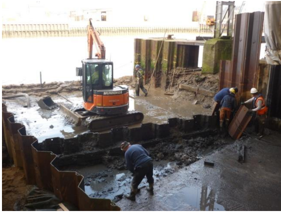
Lowering of the top of the existing tie rod wall
