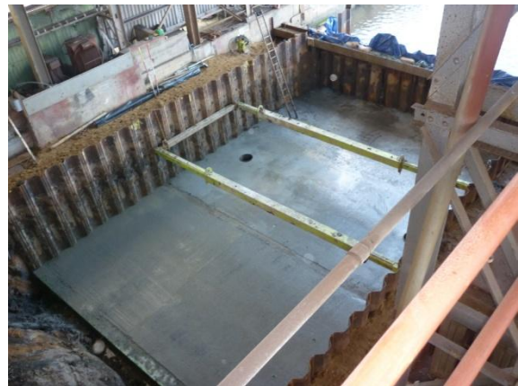
Concrete bays for dry dock being installed
