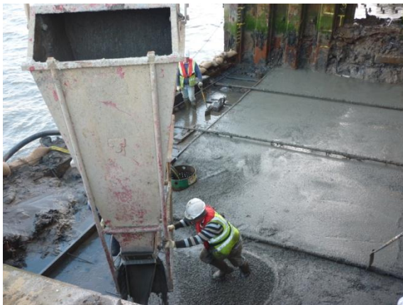
Installing concrete dock sill 300mm below Average spring low water
