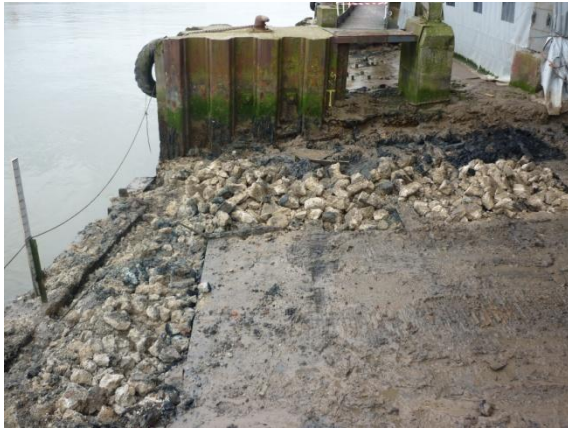
Breaking out existing concrete slip at low water
