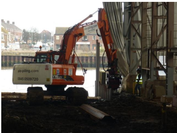
Installing sheet piled cofferdam wall
