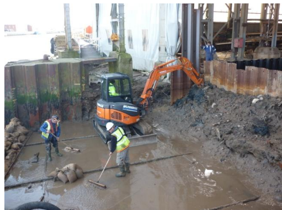
Removal of cofferdam wall
