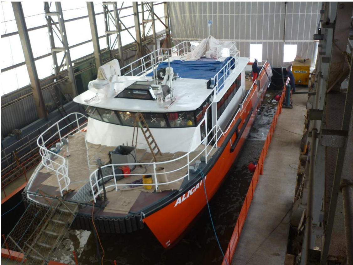
Completed mini dry dock with 1 st vessel to be launched
