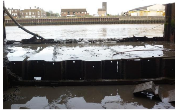
Sandbag wall being topped just after low water
