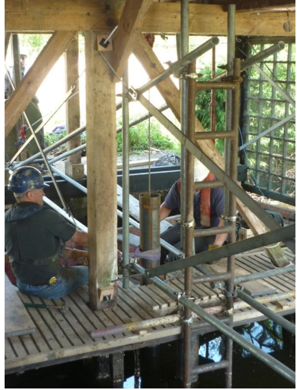
Using pulley blocks and bracing GTRP were able to install the bearing piles to a calculated set
