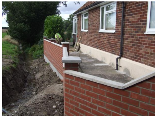
Stream back flowing down the original line
