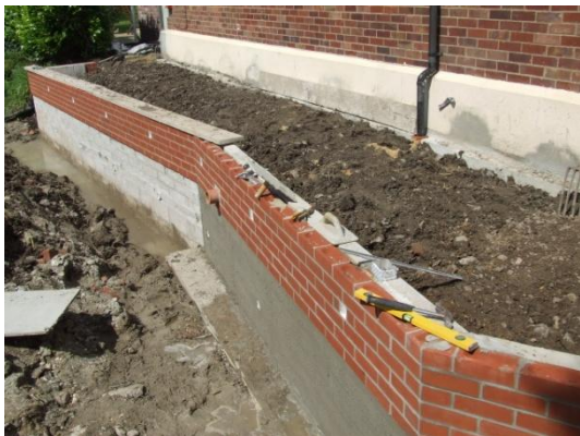
13 inch block work wall with weep holes installed
