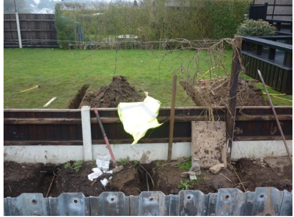
Installing tie rod system into clients neighbouring property
