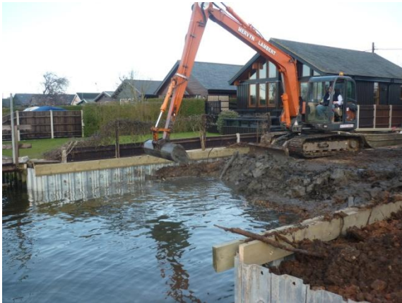
Dredging out the new boat dock
