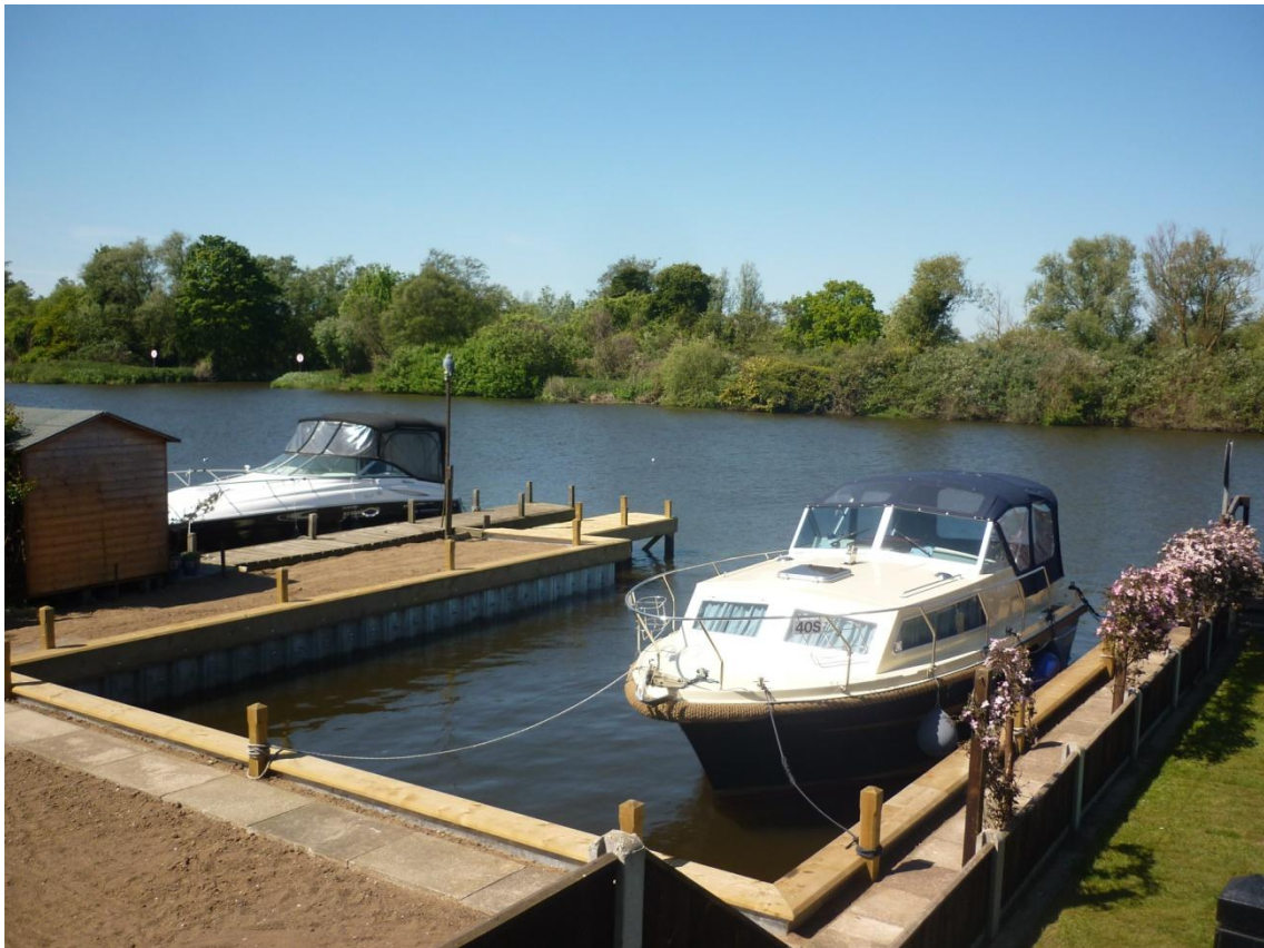
Installed boat dock landing jetty and piled foundation for new property
