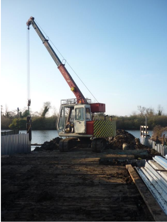
Installing 7m M11 galvanised lite piles
