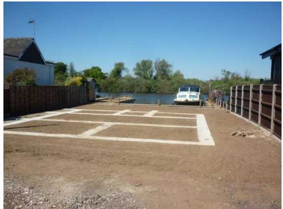
Installed piled foundations for new property
