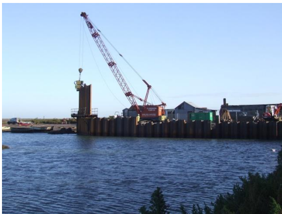
Installing sheet piled wall
