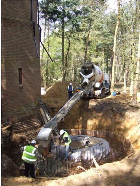
Under-pined 50% of water tower 3m below ground level
